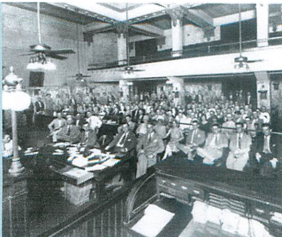
The north courtroom of the 1910 Courthouse in 1920.
